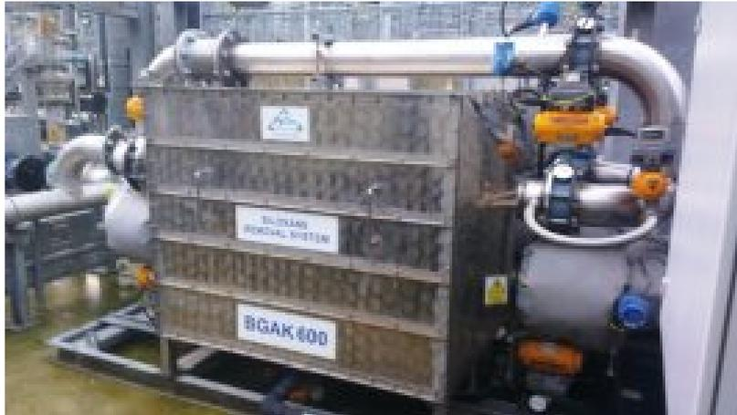
The Filters are run for a specified period of time when they are predicted to have reached their peak Siloxane loading and then the filter is switched with the 2nd clean filter. The dirty filter is now regenerated by heating it to drive off the volatile components to flare ready to be brought back on line at the end of the 2nd filter cycle.
